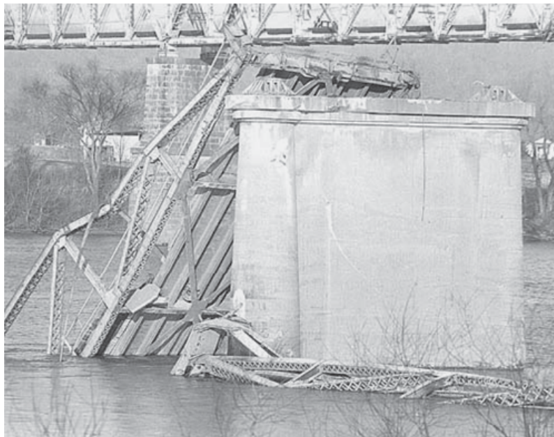
Figure 1.1: Collapse of Silver Bridge (Connor, Dexter, and Mahmoud, 2005)
